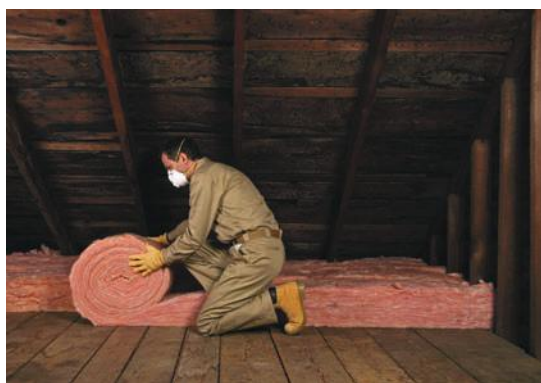
Figure 23.4b Laying lagging in a house loft
