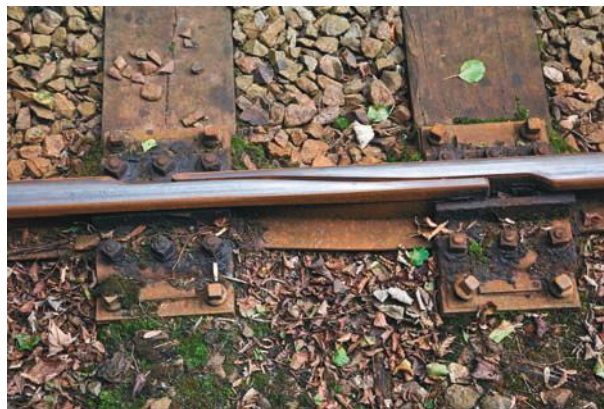
Figure 19.2a Tapered overlap of rails
