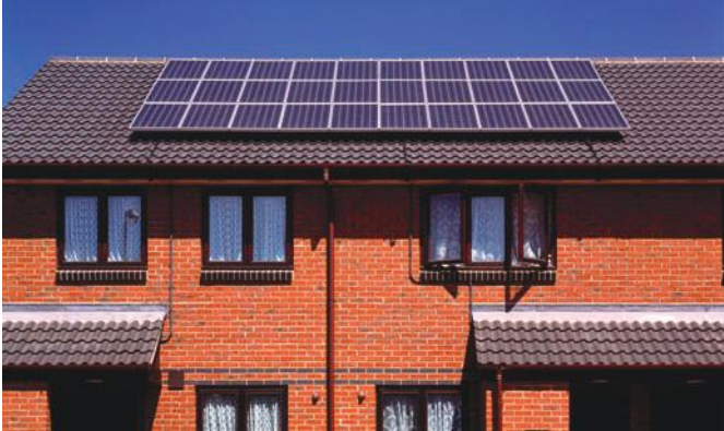
Figure 15.1 Solar cells on a house provide electricity.
